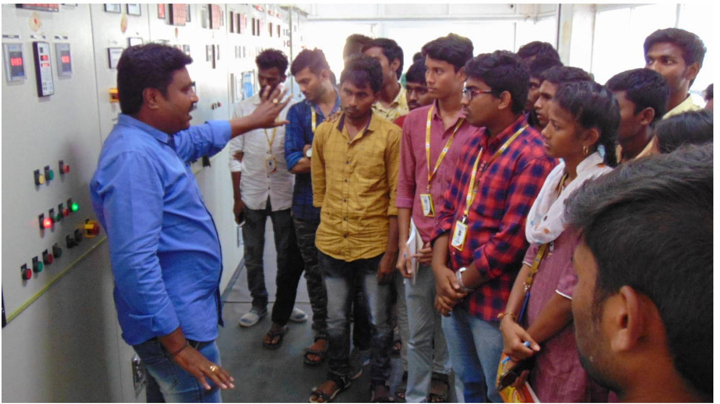
Plant A.E Briefing about controlled unit.
