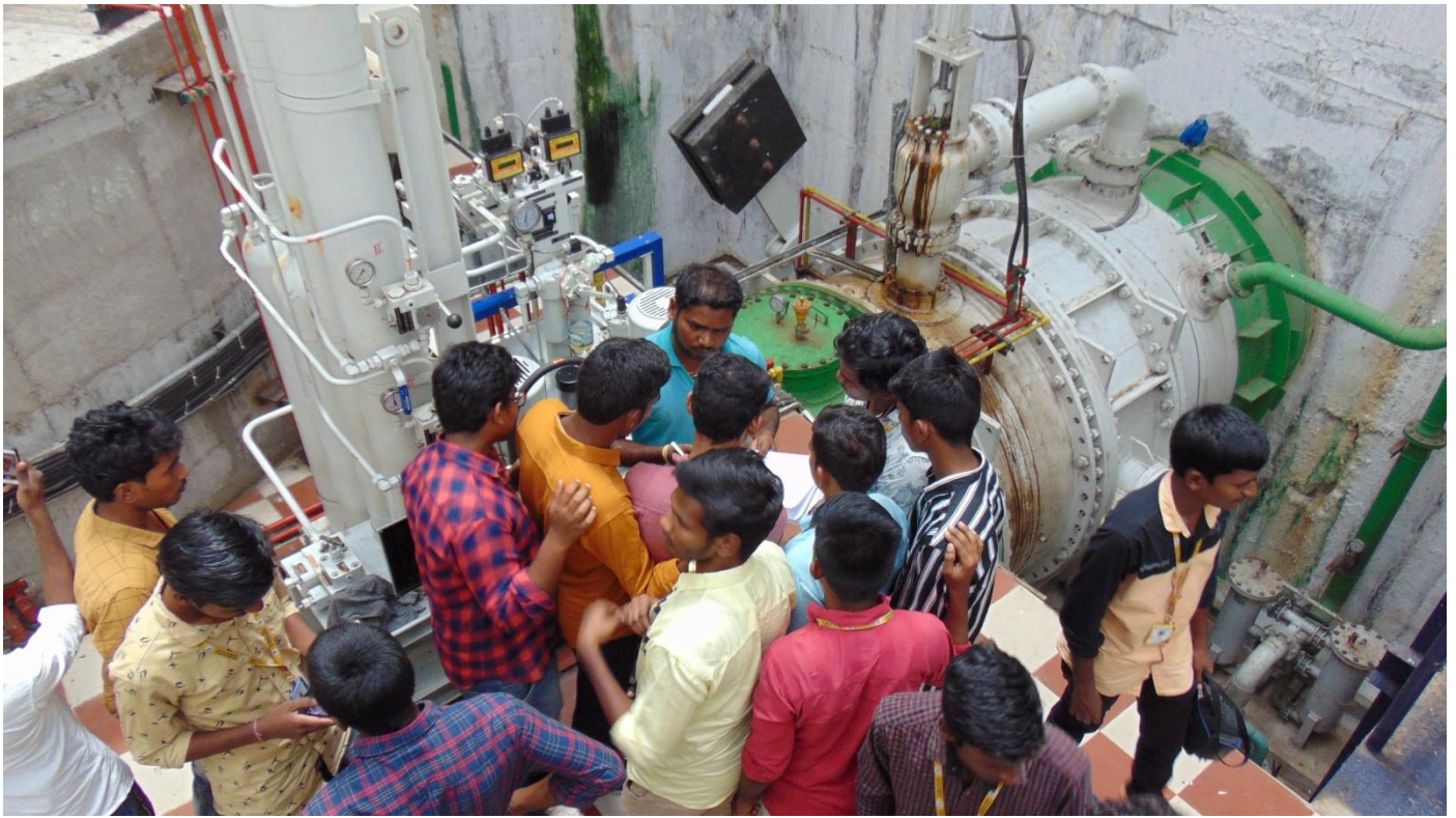
Operations Engineer Explaining about Penstock:
